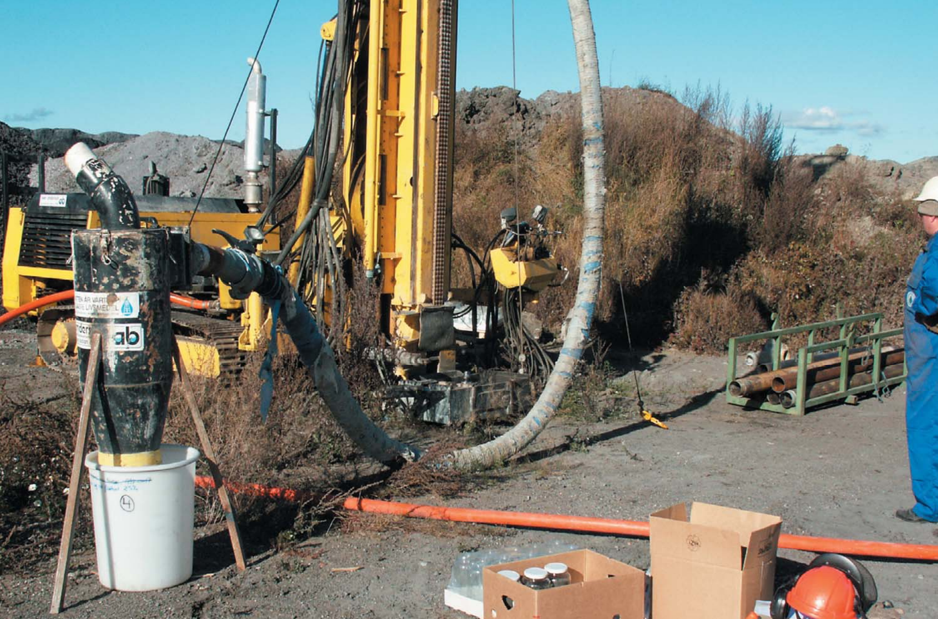
The material was collected in a drum using a cyclone. Two composite samples were taken for every meter, one of which was subsequently crushed to \leq 6 mm and homogenized
